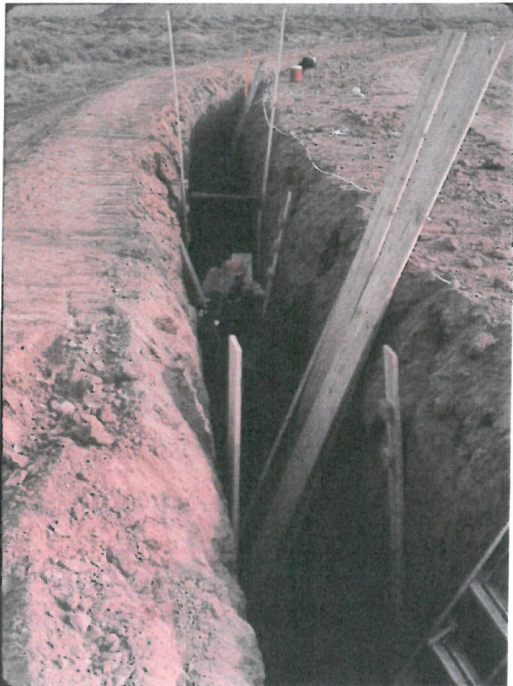
Photograph 1: Chimney drain excavation.
