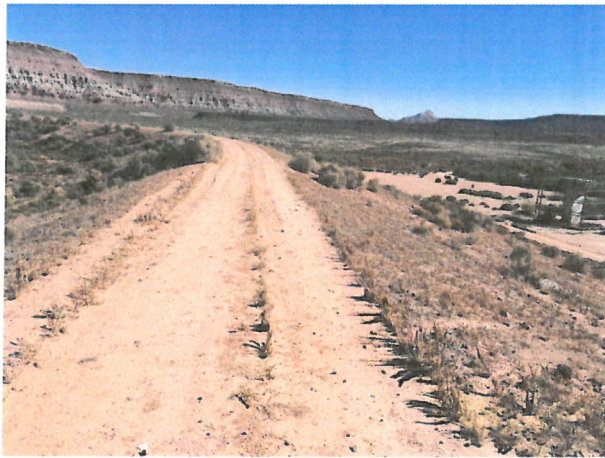
Photo D.1-14 - Looking northeast along crest of dam.
