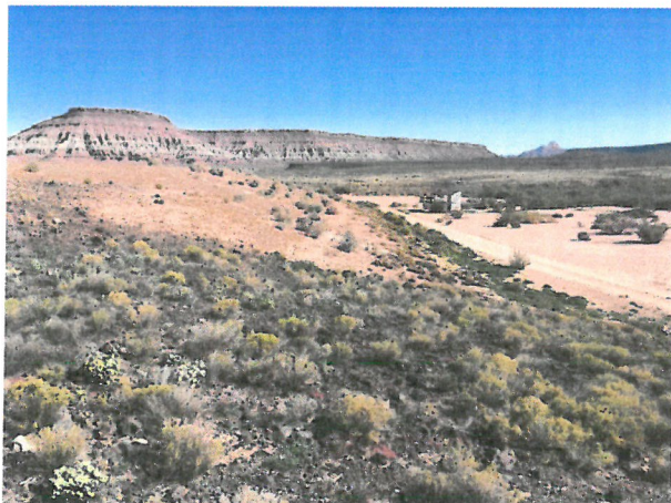
Photo D.1-10 - Looking northeast along the upstream slope of the dam.
