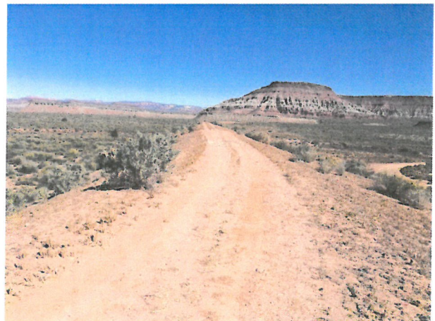
Photo D.1-23 Looking northeast along the center of the dam.
