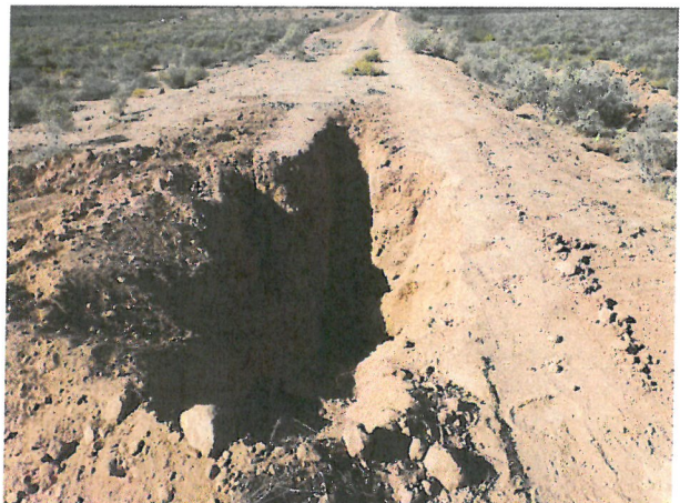
Photo D.2-A4-4 – T-10 location: Looking southwest along dam crest.
