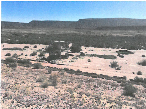
Photo D.1-4 - Looking east at discharge structure and basin.
