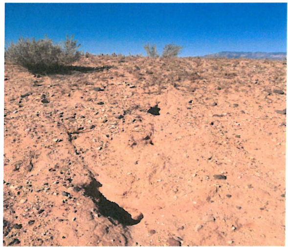
Photograph 6: Crack about 5 inches wide along upstream embankment; view to north.
