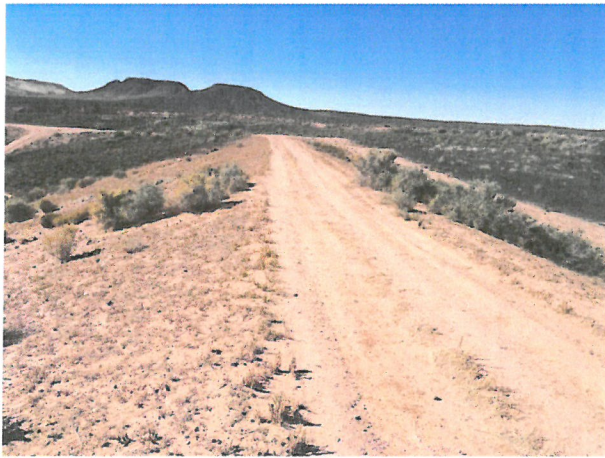
Photo D.1-20 Looking southwest along crest of dam.
