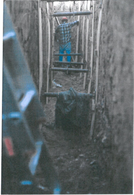
Photograph 4: Chimney drain excavation.
