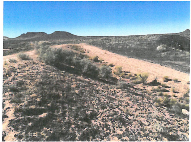
Photo D.1-21 Looking southwest along the downstream slope of dam.
