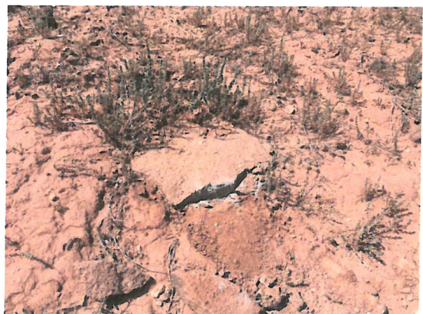
Photo D.3-54 Hole previously filled with grout.
