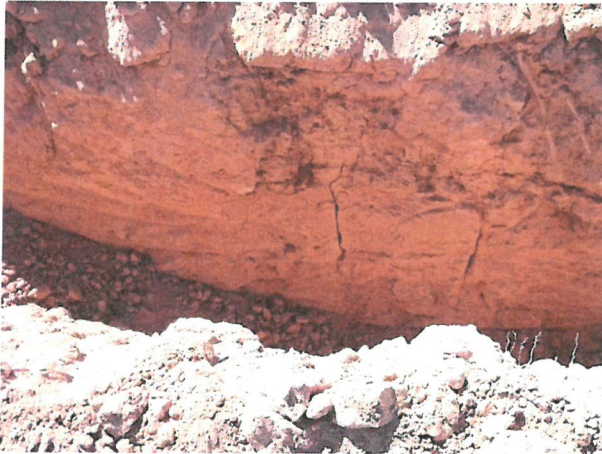
Photo D.2-A3-3 – T-7 location: Looking southeast into trench. Multiple secondary crack can be observed in southeast wall.
