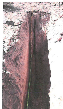
Photo D.2-A2-6 – T-6 location: Looking northwest at the transverse crack can be observed in the northwest wall of T-6.
