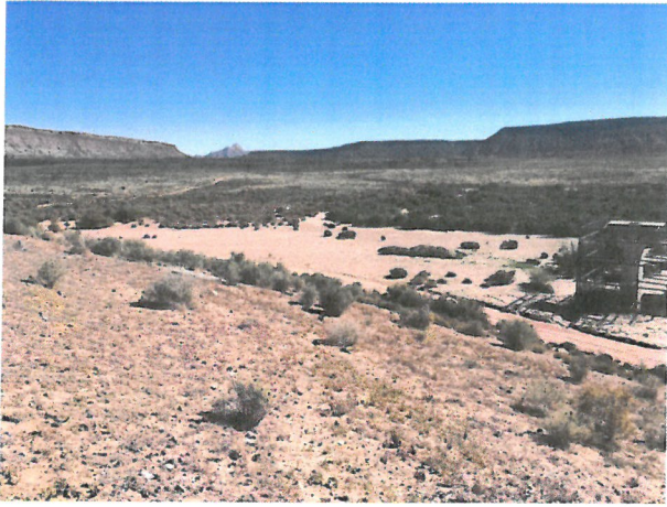
Photo D.1-6 - Looking east at discharge structure and basin.
