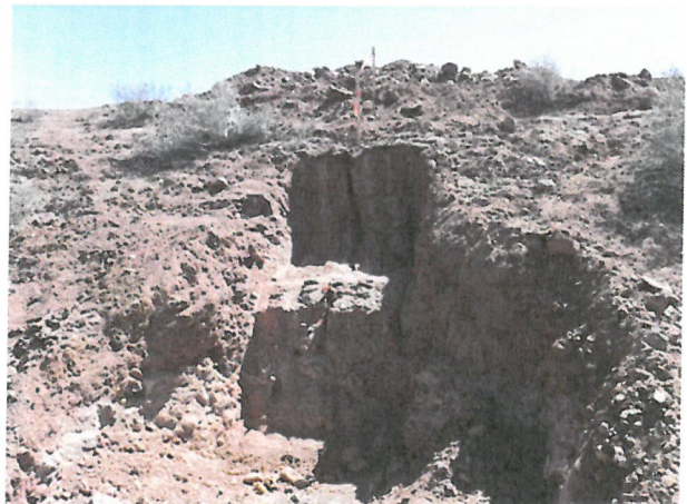
Photo D.2-A2-10 – T-15 location: Looking southeast towards T-12. One transverse crack can be observed in the upper wall and two in the lower wall of T-15. Flagged lath in the background shows the alignment with the same crack observed in T-12.
