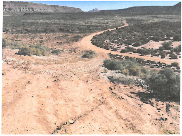
Photo D.1-31 Vehicle tracks climbing up dam on upstream slope.
