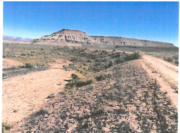
Photo D.1-15 - Looking northeast along the downstream slope of the dam.
