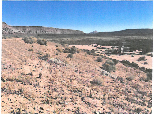
Photo D.1-13 - Looking northeast along the upstream slope of the dam.
