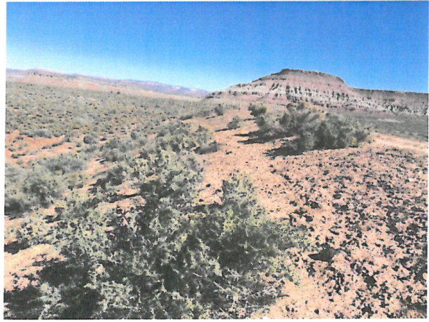
Photo D.1-25 Looking northeast along the downstream slope of the dam, knee-high vegetation.
