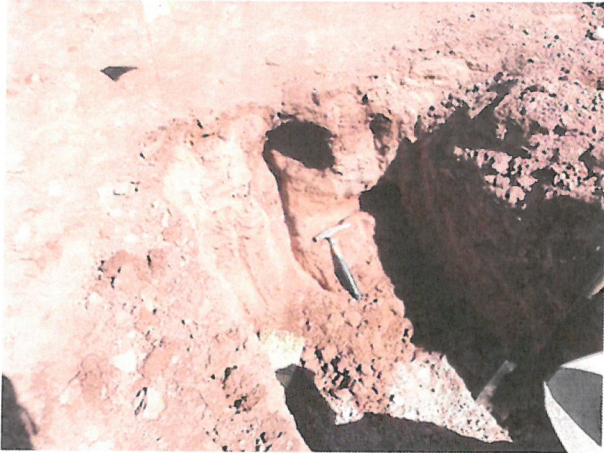
Photo D.2-A4-7 – T-11 location: Looking north after 36 inches of excavation at H-20. Transverse crack can be observed in northwest wall.
