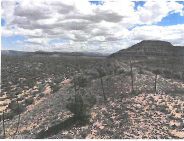
Photo D.1-30 Looking northeast along the upstream slope of the dam, fence crossing dam.
