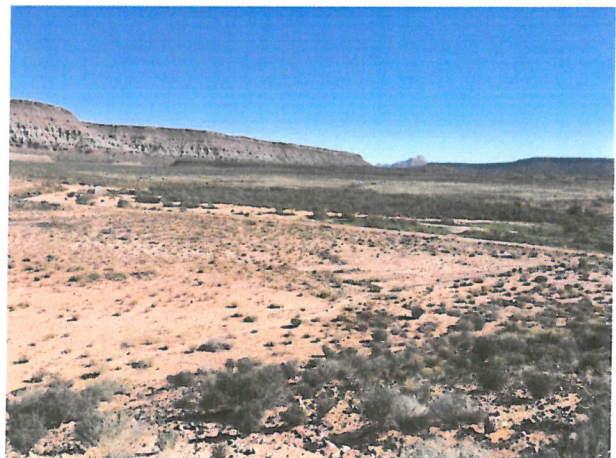
Photo D.1-9 - Looking east at emergency spillway.
