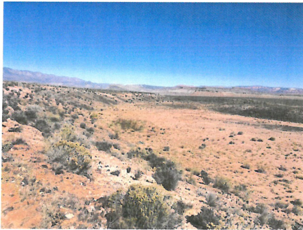
Photo D.1-8 - Looking north, at emergency spillway.
