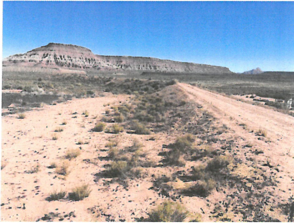
Photo D.1-12 - Looking northeast along the downstream slope of the dam.
