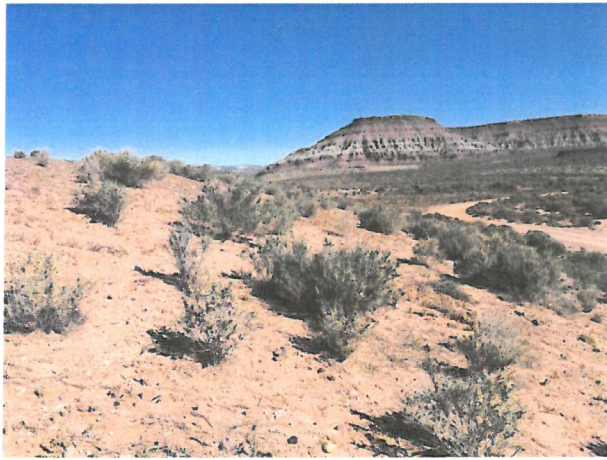
Photo D.1-24 Looking northeast along the upstream slope of the dam.
