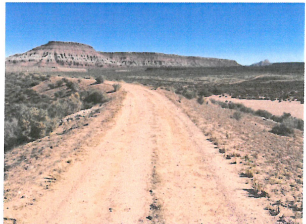
Photo D.1-17 Looking northeast along crest of dam
