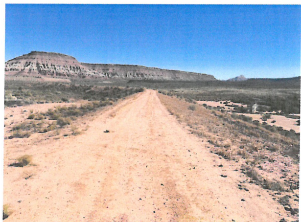
Photo D.1-11 - Looking northeast along crest of dam.
