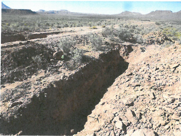
Photo D.2-A4-3 – T-9 location: Looking south after exploration.
