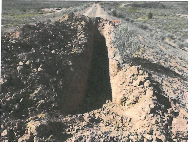
Photo D.2-A3-1 – T-7 location: Looking southwest along dam crest.
