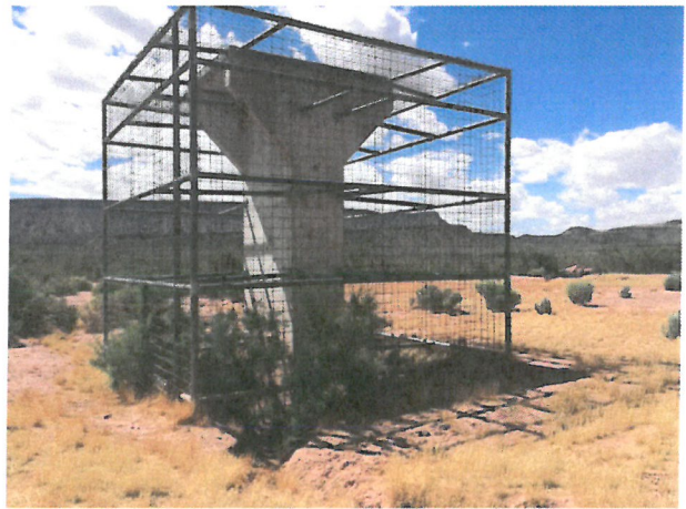
Photo D.1-33 Northwest face of drainage structure, vegetation in cage.
