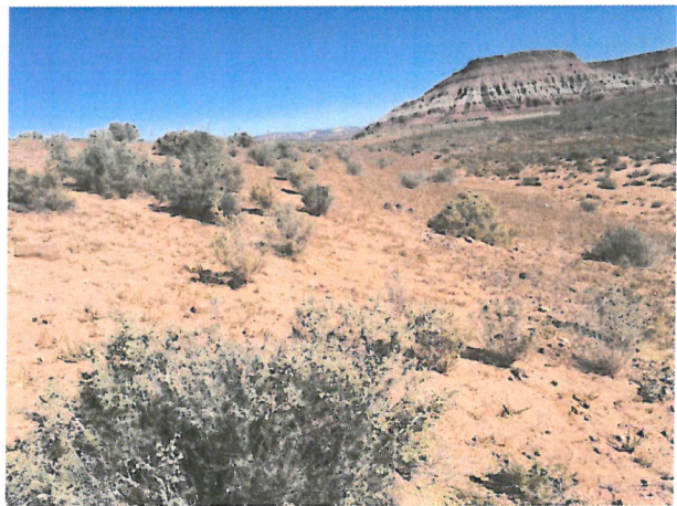
Photo D.1-27 Looking northeast along the upstream slope of the dam.
