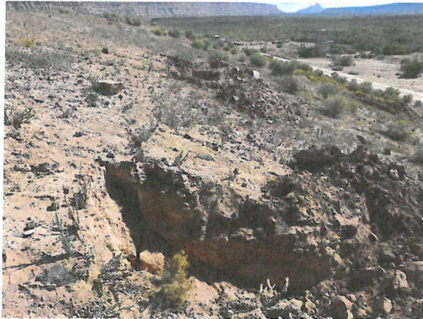
Photo D.2-A1-3 – Overlooking Area 1. Looking northeast along the upstream slope of dam showing T-1 (foreground) in relation to T-2, T-3 and T-4 (background).
